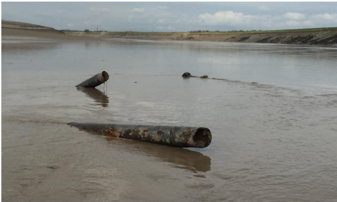
Pawlett Hams supply pipeline failure after embankment slip in Oct 2015
