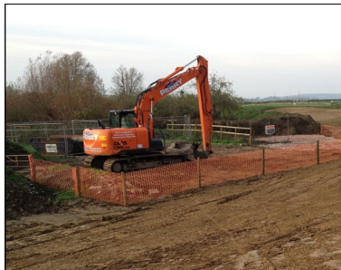
Work in progress at Thorney Ring Bank
