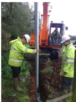
Piles being inserted at Henley Corner, Kings Sedgemoor
