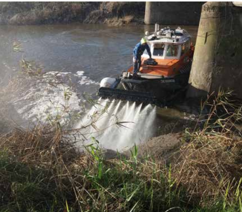
De-silting operations at Blake Bridge in Bridgwater
