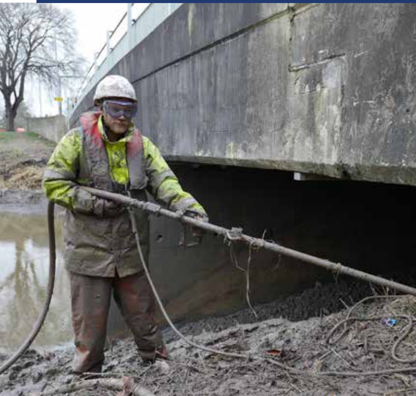
De-silting operations at Blake Bridge in Bridgwater
