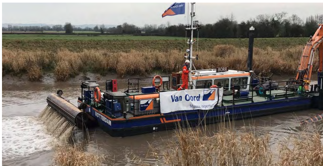
Figure 3. The BORR with the WID T-pipe pumping but elevated above the water surface.
