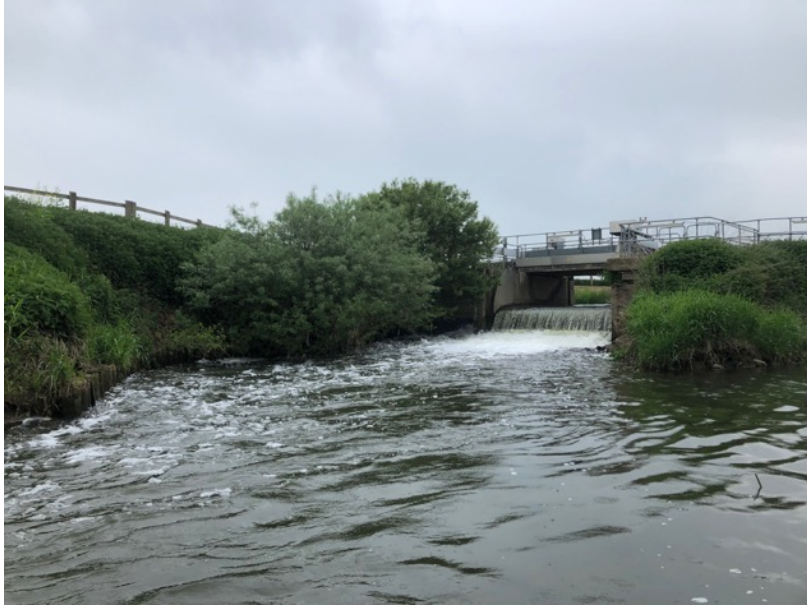
Plate 2: Freshwater flow over control structure at Oath Lock creating attractant flow to support fish passage upstream
