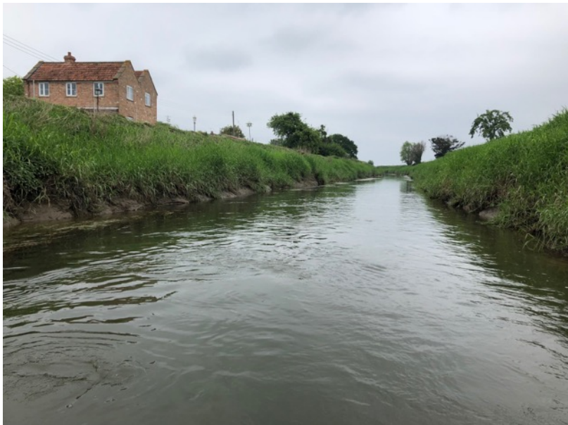
Plate 3: Typical view showing re-sectioned and re-aligned planform, influence of tide on water levels, smooth flow, no in-channel habitat/features from trees
