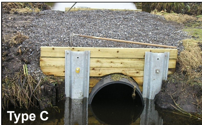
Timber and trench sheet headwall (with tie bars)
