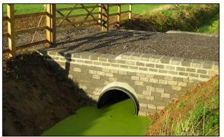
Height of wall to invert <1m = wall thickness must be 225mm (9") Height of wall to invert >1m = wall thickness must be 460mm (18") Both walls to be battered back by 25mm per block rise.
