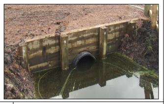
Steel (motorway barrier) Headwall
